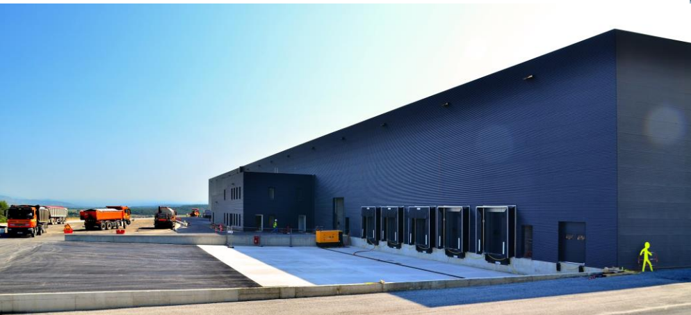
Large Storage Facility
